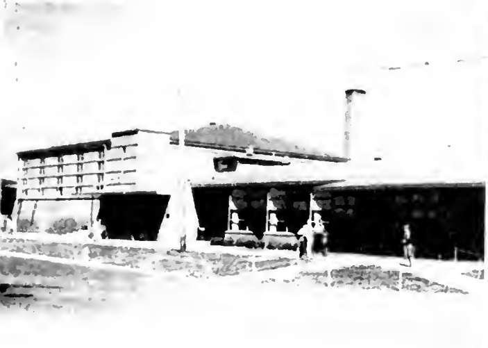
Henry J. Kaiser Company photograph Each school has its library, gymnasium and assembly hall
